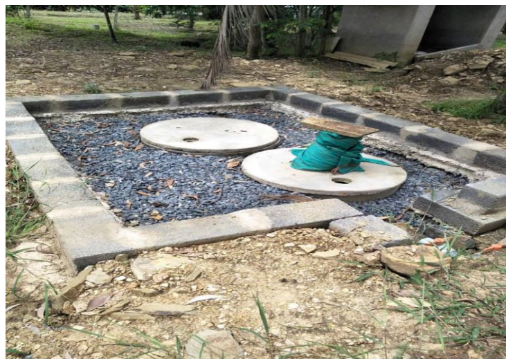
Ring model rainwater harvesting structure
